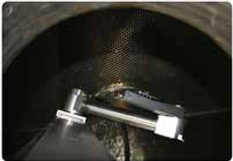
Inspection Services for Steam Generator Tubes (ECT)
